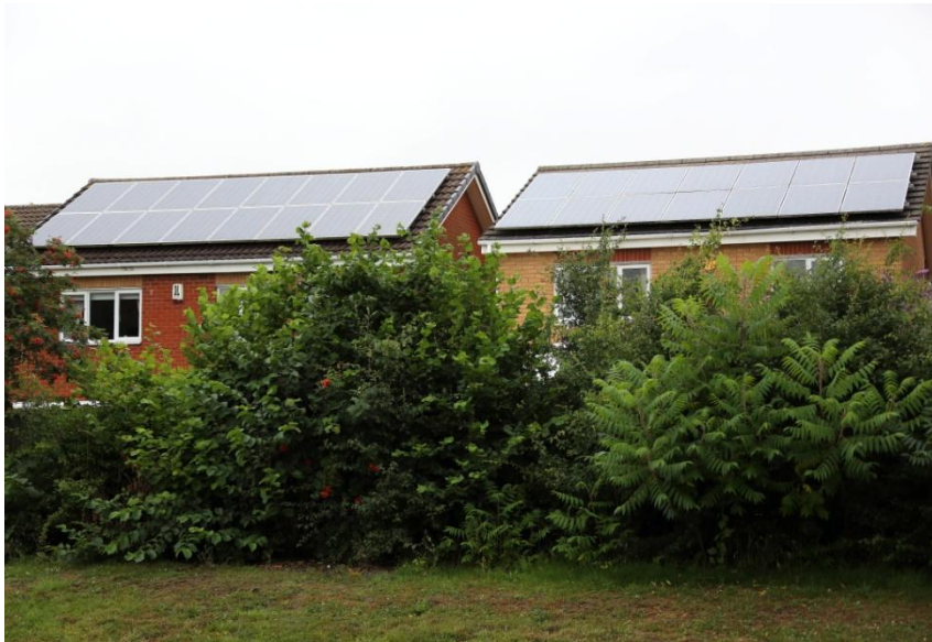
South facing roofs with solar panels
