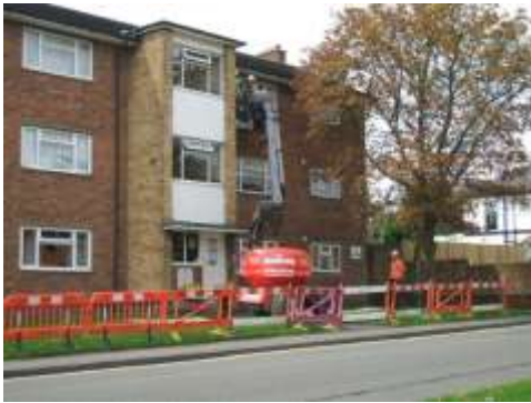
Gutter clearing by local builders, Harvey & Clarke
