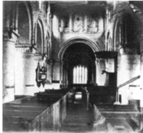
This is the only known photograph of the interior of the parish church prior to its restoration in 1859-60. Courtesy of Philip Heath.
