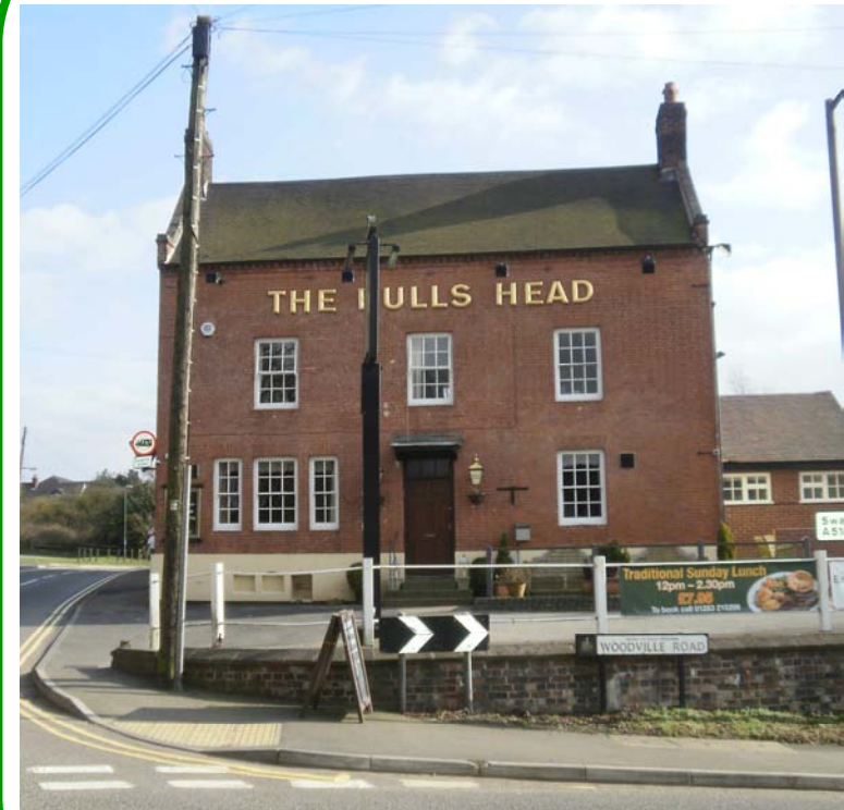
The Bulls Head, Hartshorne which is a listed building
