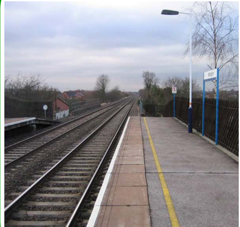
Willington Train Station
