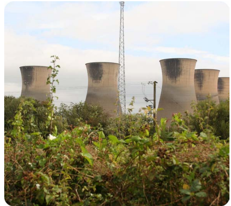
View of former power station cooling towers from the Trent Mersey Canal towpath
