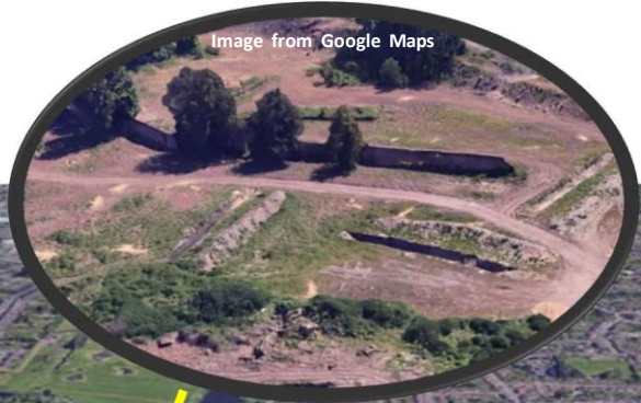
Grade II listed garden wall to east of sunken gardens at site of Drakelow Hall
