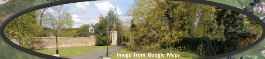
Grade II listed gate piers and adjoining walls at Drakelow Lodge
