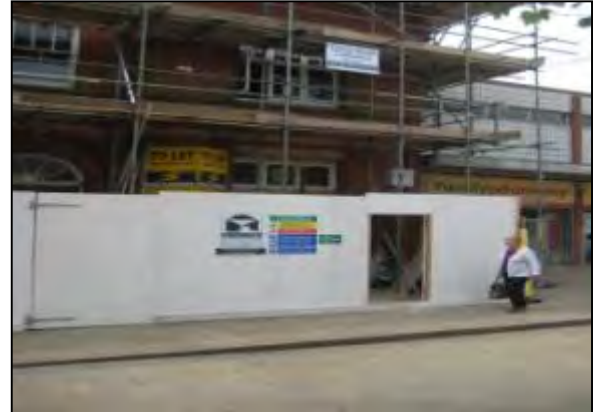
Photograph (bottom right): Vacant building under refurbishment at 4 High Street
