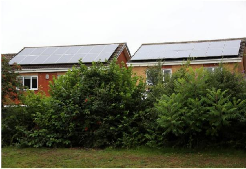
South facing roofs with solar panels
